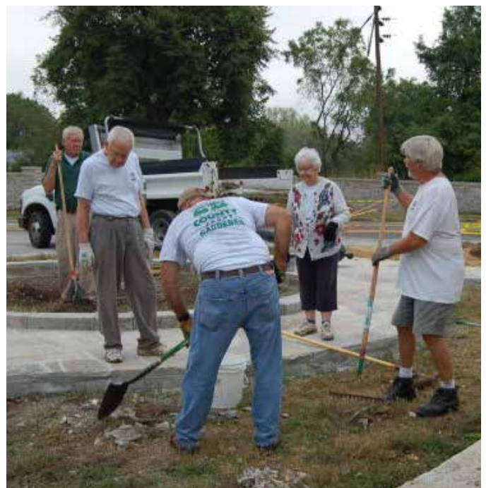
Work on the Jefferson Barracks Gateway
